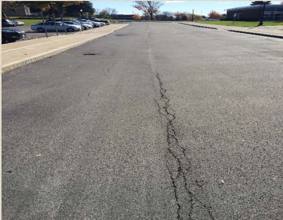
PAVEMENT (ROADWAYS & PARKING LOTS)
