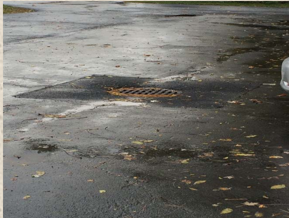
CATCH BASINS DROP INLETS/MANHOLES
