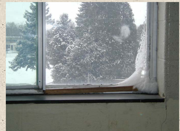
WINDOW SYSTEM ORIGINAL SINGLE GLAZED WITH MINIMAL INSULATED PANEL
