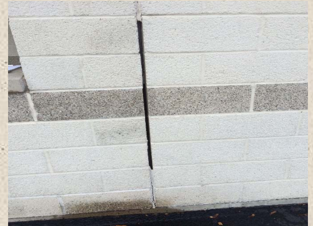
REPOINT MASONRY & RESEAL WINDOW/DOOR PERIMETERS
