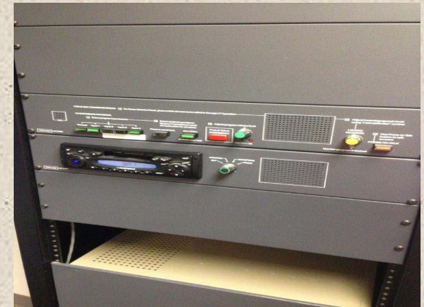
PA & CLOCK SYSTEM REACHED END OF USEFUL LIFE. PHONE IS ANALOG
