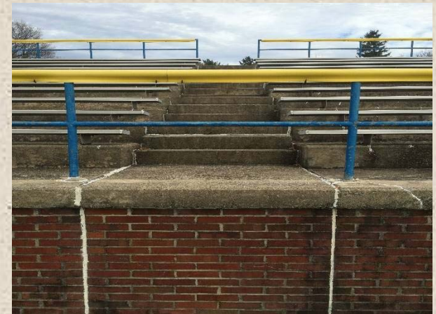
REPAIR & RECONSTRUCT CONCRETE BASE, REPOINT MASONRY AS REQUIRED
