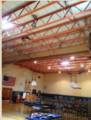
INSTALL DAYLIGHT CONTROLS IN CLASSROOMS & REPLACE AUDITORIUM/STAGE, KITCHEN & GYM LIGHTING WITH LED
