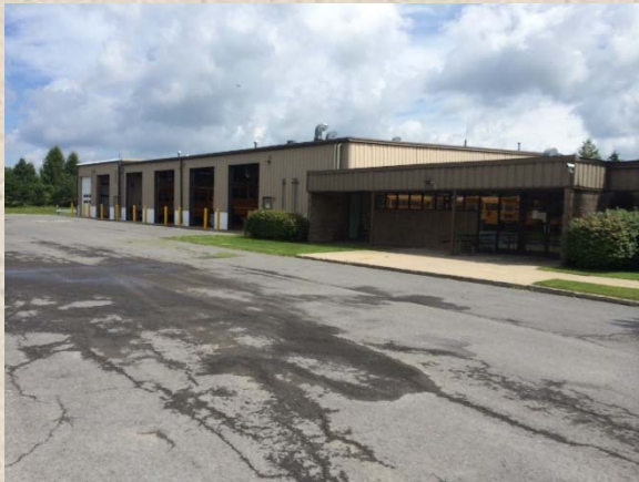
PAVEMENT (ROADWAYS & PARKING LOTS)
