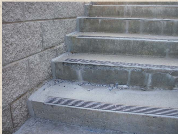
EXTERIOR STEPS, STAIRS, AND RAMPS
