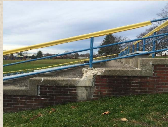
CONCRETE & BRICK BLEACHER STRUCTURE & METAL HANDRAILS
