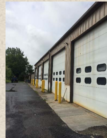
PAVEMENT, STEPS, AND RAMPS
