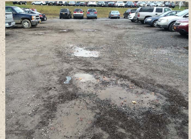
PAVEMENT (ROADWAYS AND PARKING LOTS)
