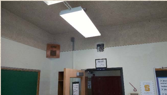
REPLACE PA & CLOCK SYSTEM. PHONE CHANGE TO DISTRICT WIDE VOIP SYSTEM
